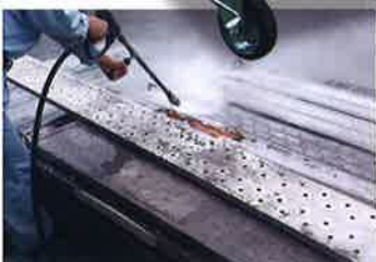
架設足場洗浄
